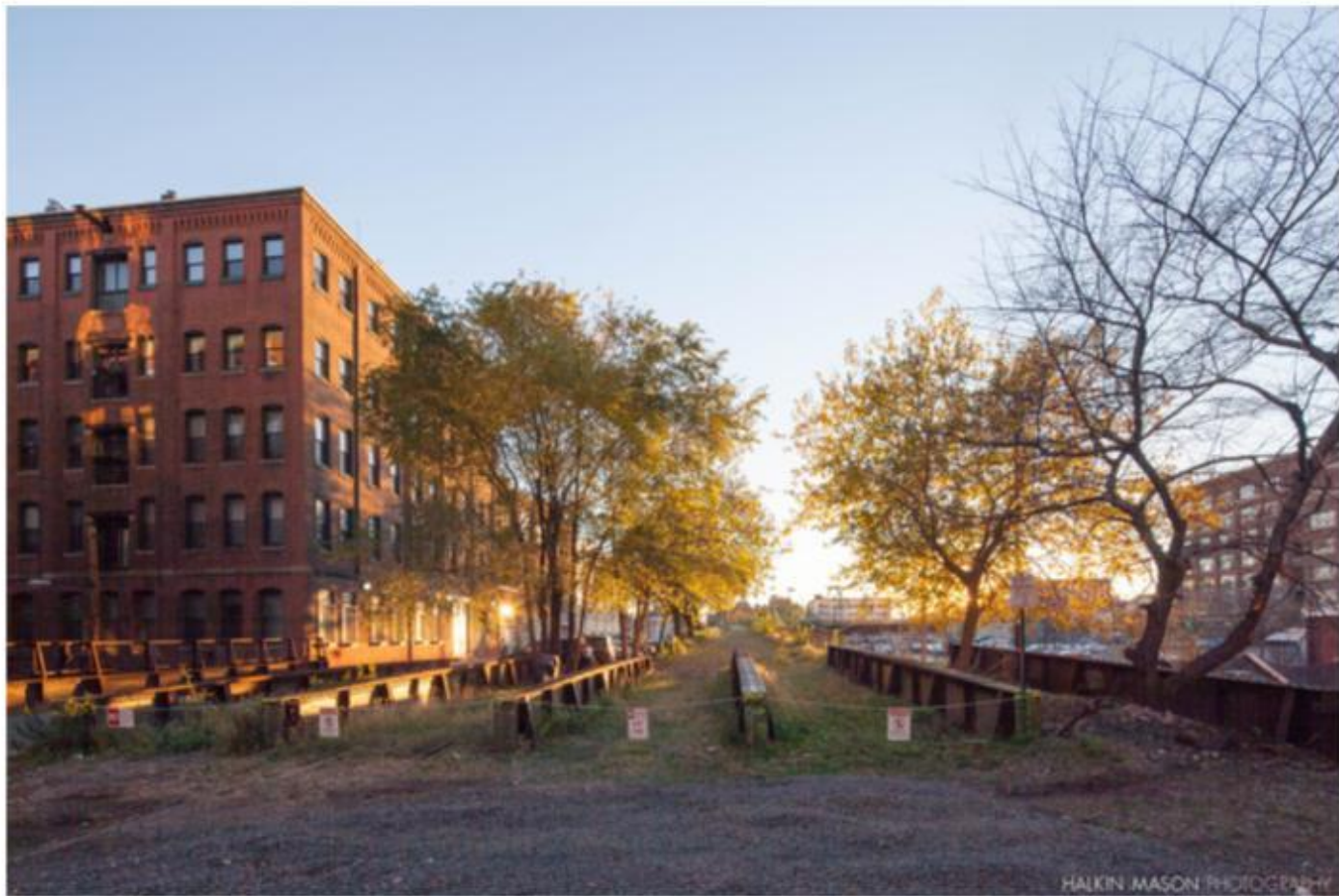
Before view of Phase I of the Rail Park.
