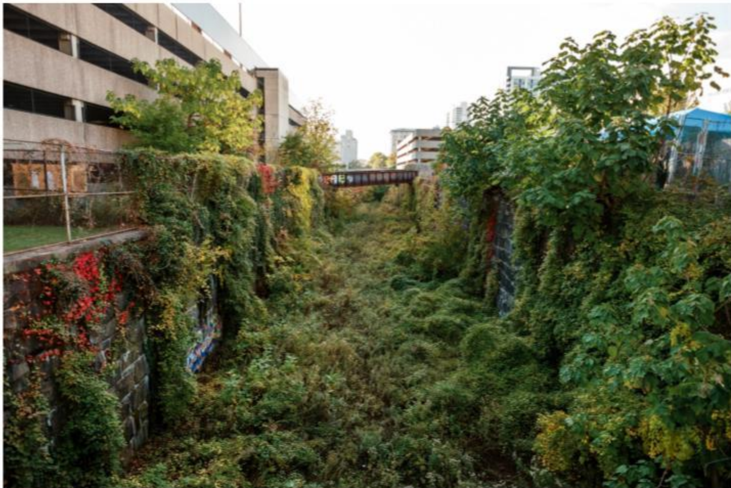
Current state of Phase II site (The Cut).
