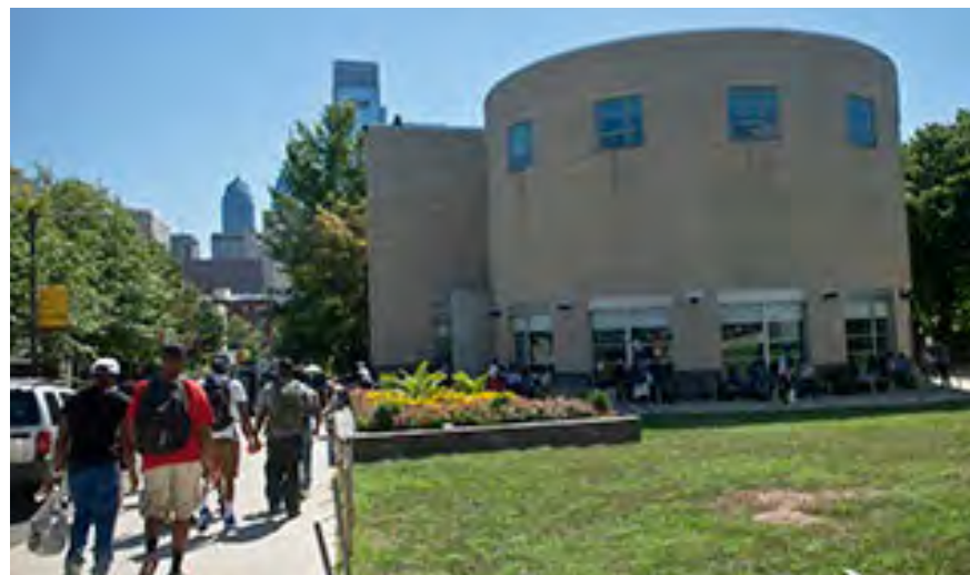
Winnet Building Entrance facing 17th Street
