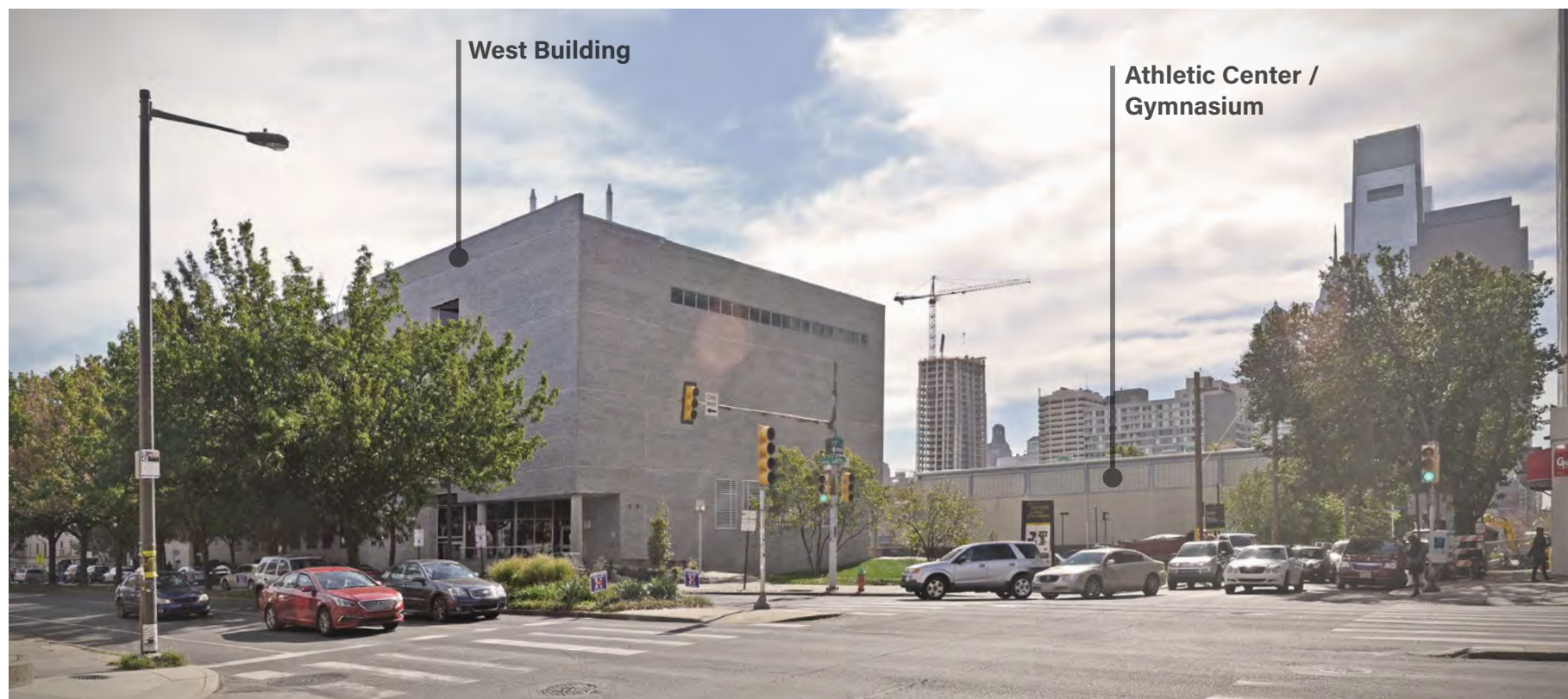
West Building and Athletic Center Existing view of 18th and Spring Garden Streets corner looking South
