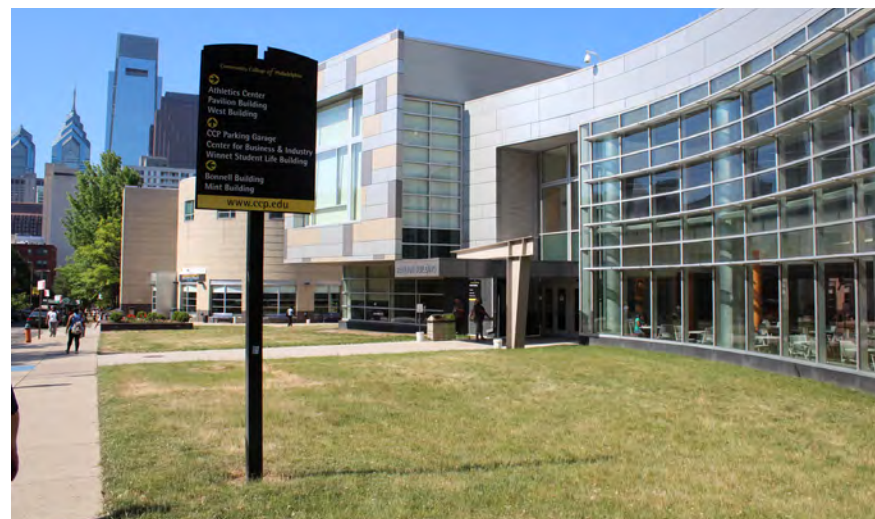
Pavilion Building Pavilion Building entrance off 17th Street
