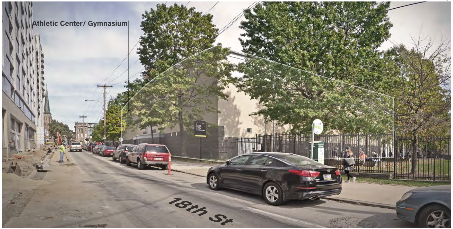
Gymnasium / Athletic Center View of Gymnasium / Athletic Center along 18th Street
