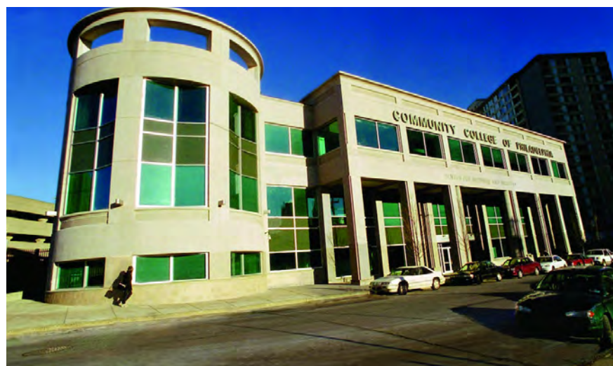
Center for Business and Industry (CBI) Building Main entrance along 18th Street
