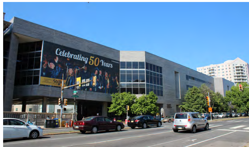
West Building West Building along Spring Garden Street
