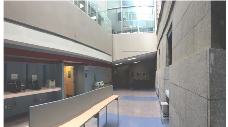
Existing light well at Bonnell Building
